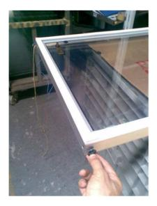
9. Put together the cables with adhesive tape to make it easier to put these through the door.
